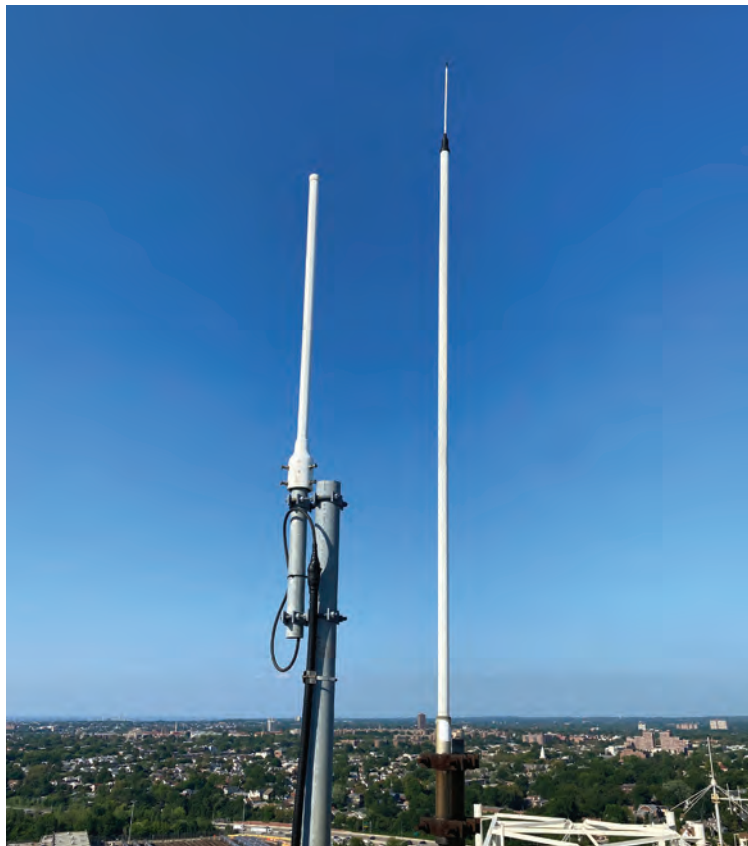
LiveATC feed equipment must be within line of sight of airport facilities and local traffic to capture radio calls.
