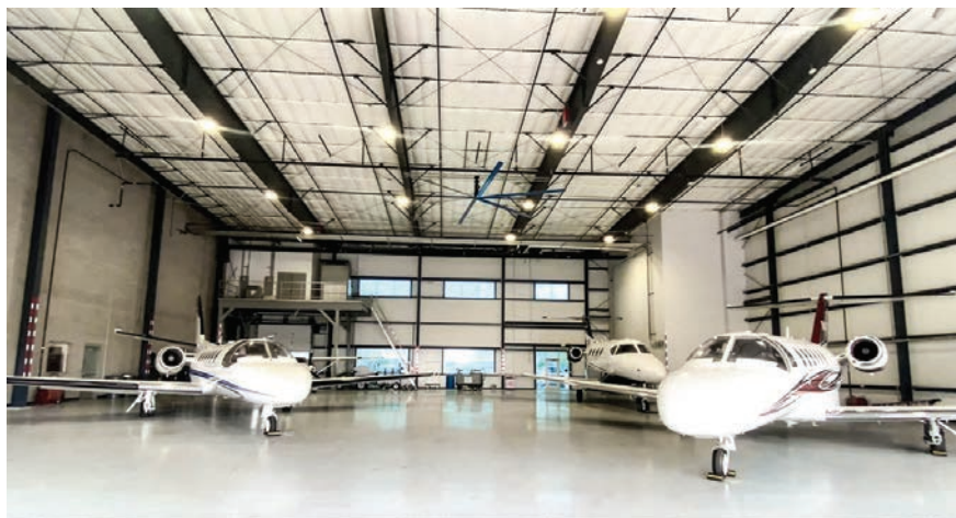
Cunningham Aviation has 60,000 sq ft of aircraft storage space at KFFZ, including a 12,000-sq-ft hangar that can accommodate the latest ultra-long-range business jets.
