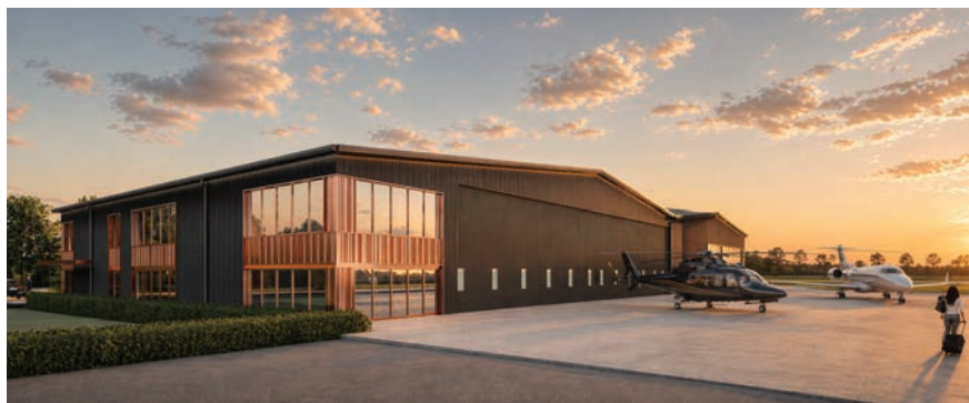
New hangars and a terminal are part of a $20 million modernization project at EGLK.
