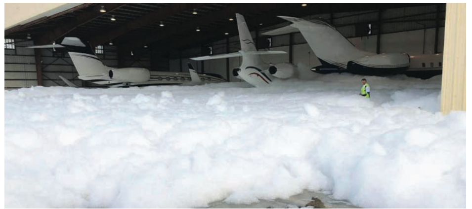
With the 2022 revision to NFPA's Standard on Aircraft Hangars easing the requirements for hangar fire foam systems in Group II hangars, costly accidental discharge events may end.
