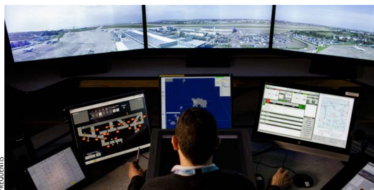
Jersey Airport's remote tower has demonstrated capability to handle up to 32 movements per hour.
