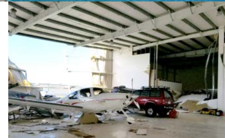
At Naples Municipal Airport nearly every hangar sustained some damage. At least six hangars are either substantially damaged or destroyed. The structures shown belong to Naples Jet Center, which reported that the water receded the day after these photos were taken.
