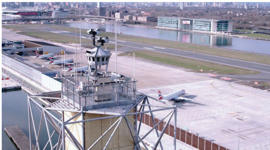
Aircraft landing and taking off from London City Airport are now remotely managed from an air traffic management facility 72 miles away.
