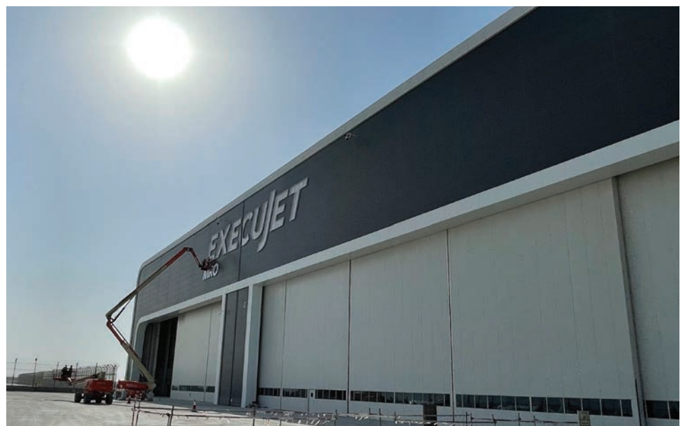
ExecuJet’s new MRO facility at Al Maktoum International Airport is designed to accommodate the largest business jets, including Dassault’s upcoming 6X and 10X, as well as jets from other manufacturers.
